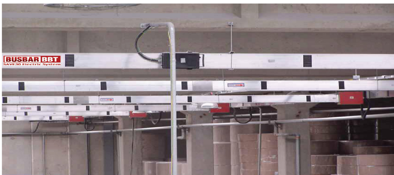
Standard Power Busbar Elements
