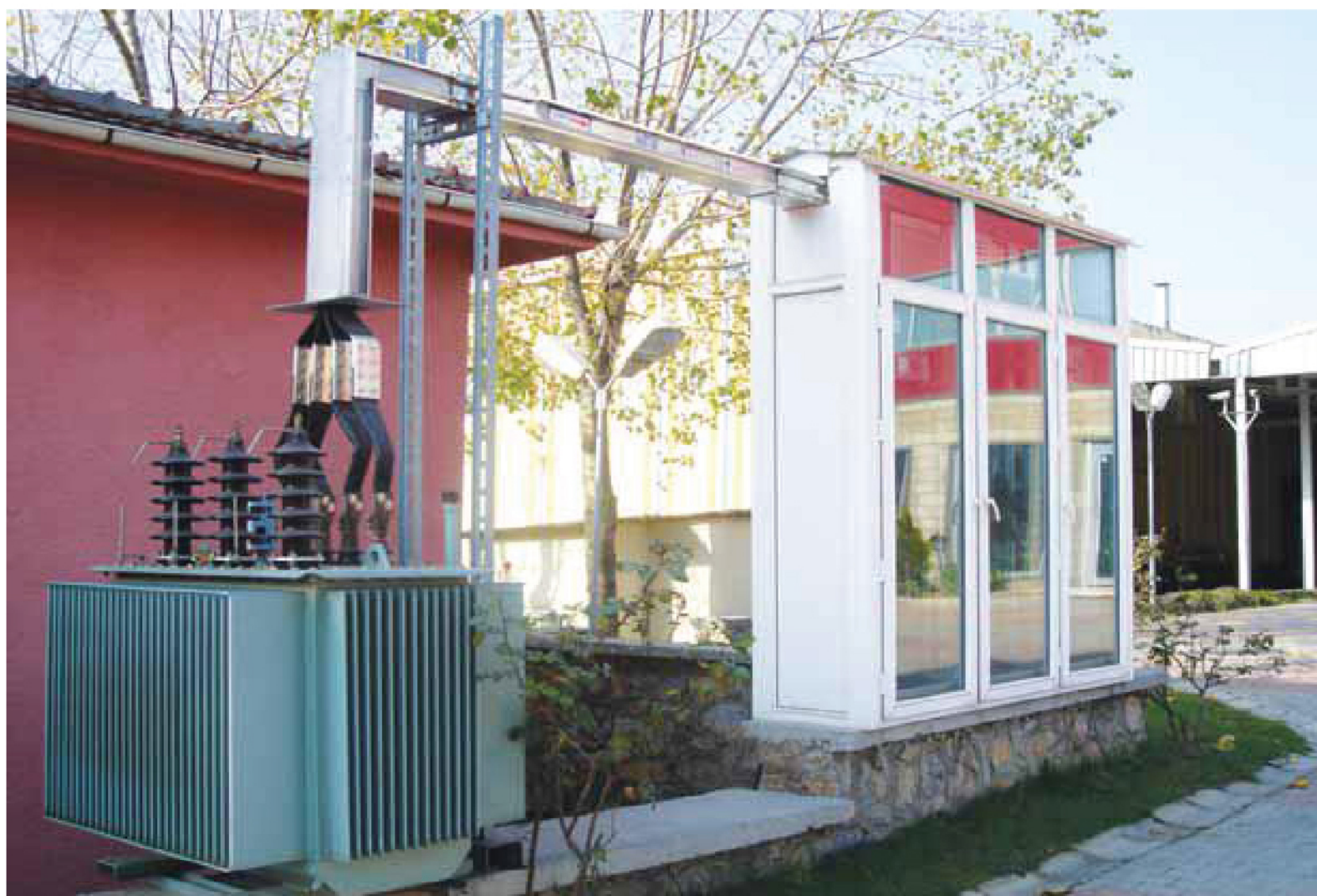
Standard Busbar Elements Connected With The Substation
