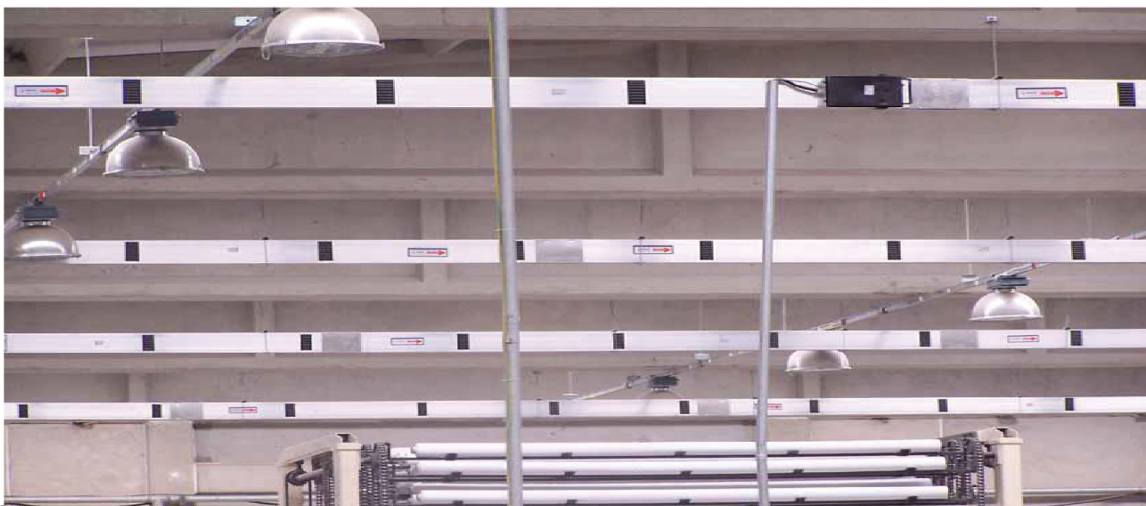
Standard Lighting Busbar Elements
